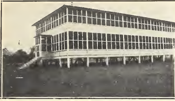
FIG. 8. Compania Agricola de Ulua, La Lima, Republic of Honduras. A well-screened house built by the United Fruit Company for bachelor quarters.
